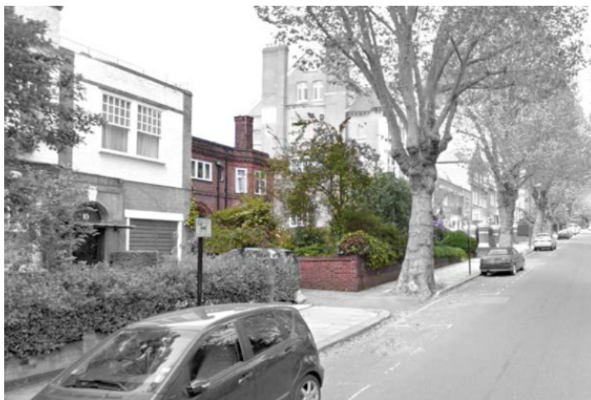
Photograph 1: View of 10a looking north-east from Heath Drive. (Image courtesy of Google Maps)
