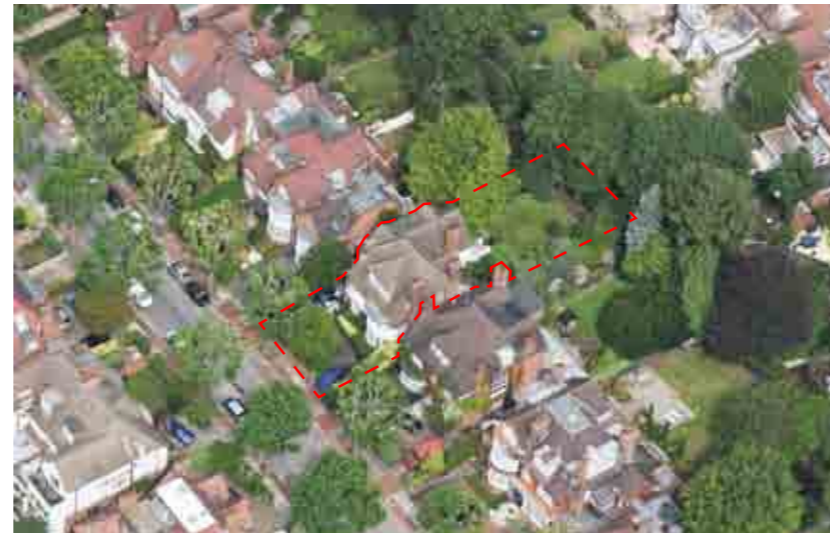
AERIAL VIEW NORTH.
