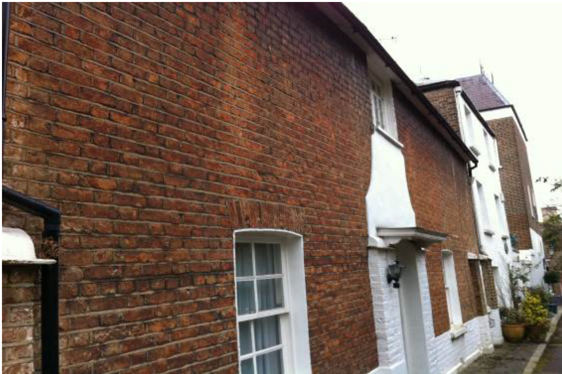
Close up of front elevation.
