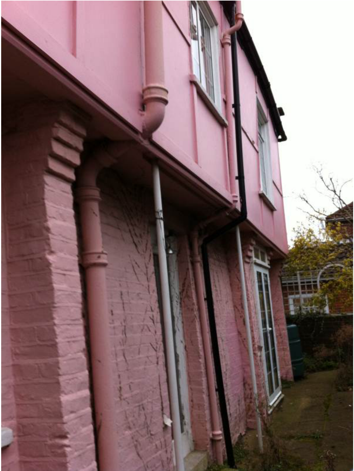
View of rear elevation.
