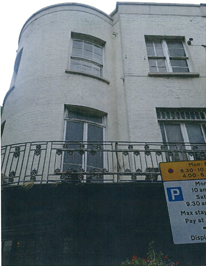
Photograph 2 – Left side Parkway Elevation
