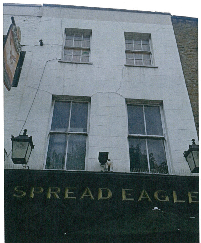
Photograph 3 – Right side Parkway Elevation
