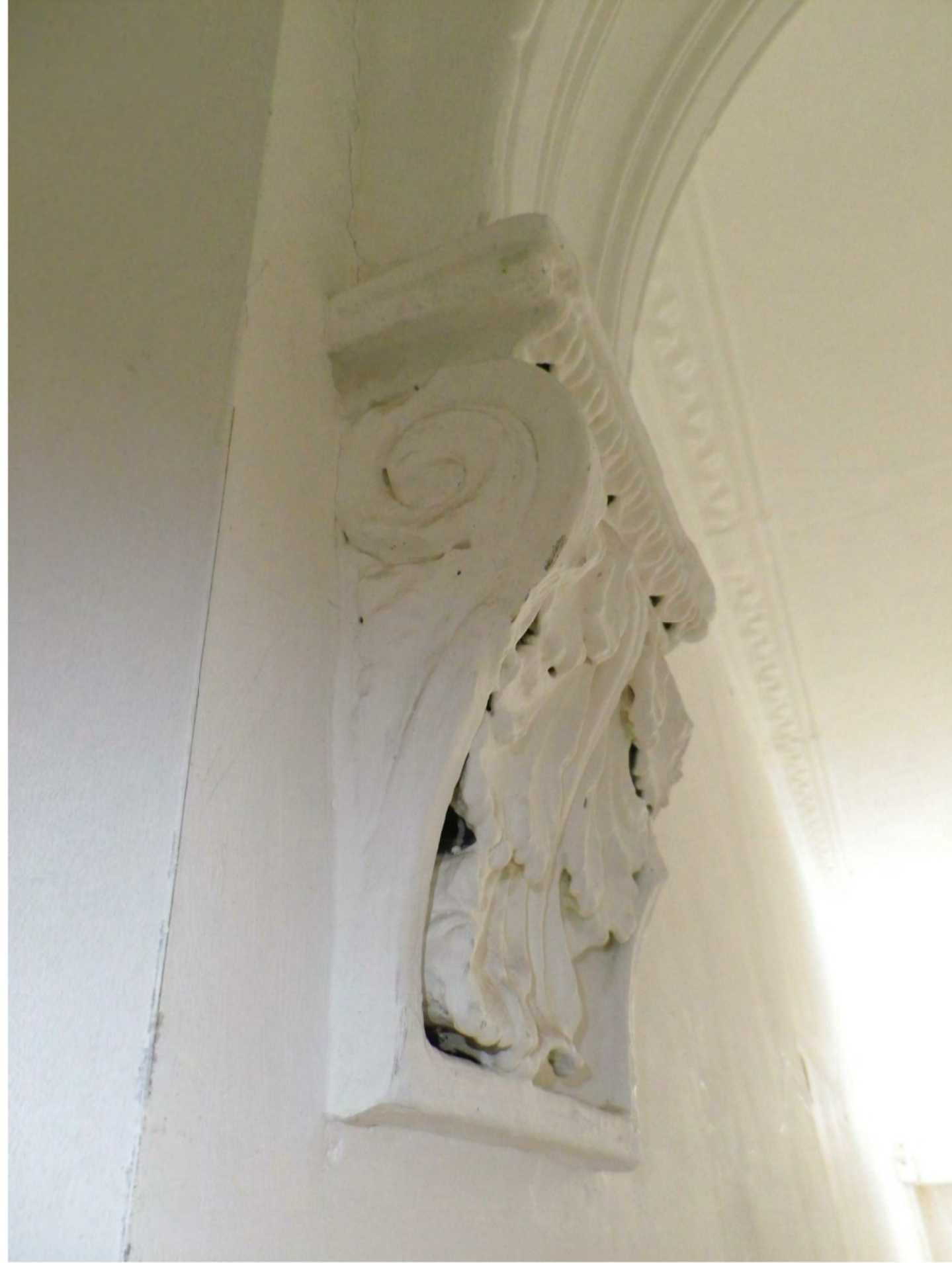
Archway and moulding in hall to be retained
