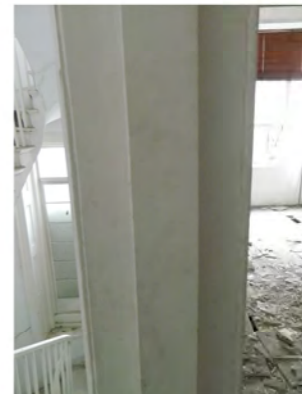
DH-01 View of door frame on 1st floor landing
