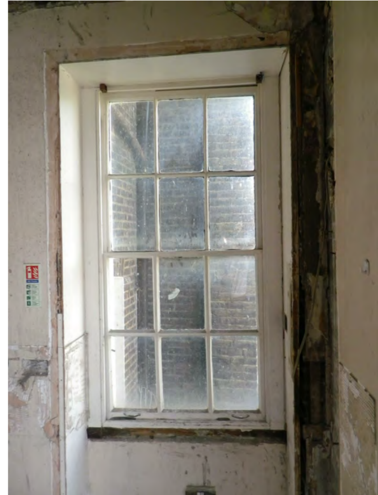
2nd floor rear side window
