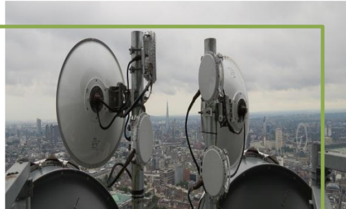
Image 6.3 - Rooftop View of 0.6m
