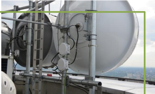
Image 6.2 - Rooftop View of 1.8m
