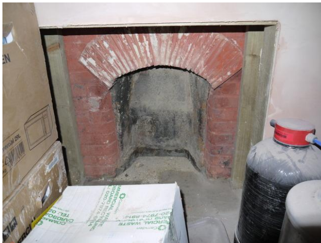
Fireplace surround with projecting creasing tile arch and bull-nosed brick jambs
