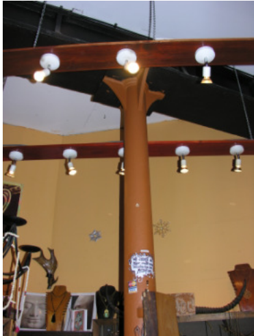
Figure 15: Cast iron column and girder south end interior
