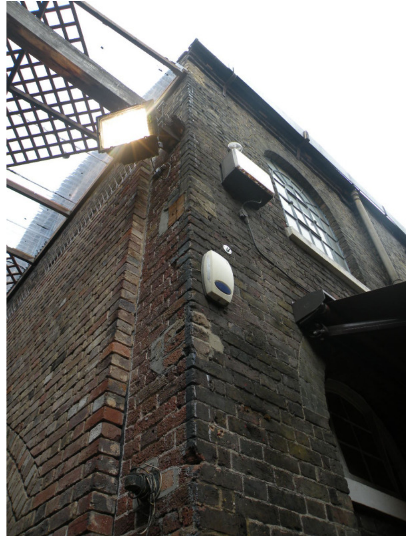
Figure 11: Tack Room south east corner showing overlapping brickwork.
