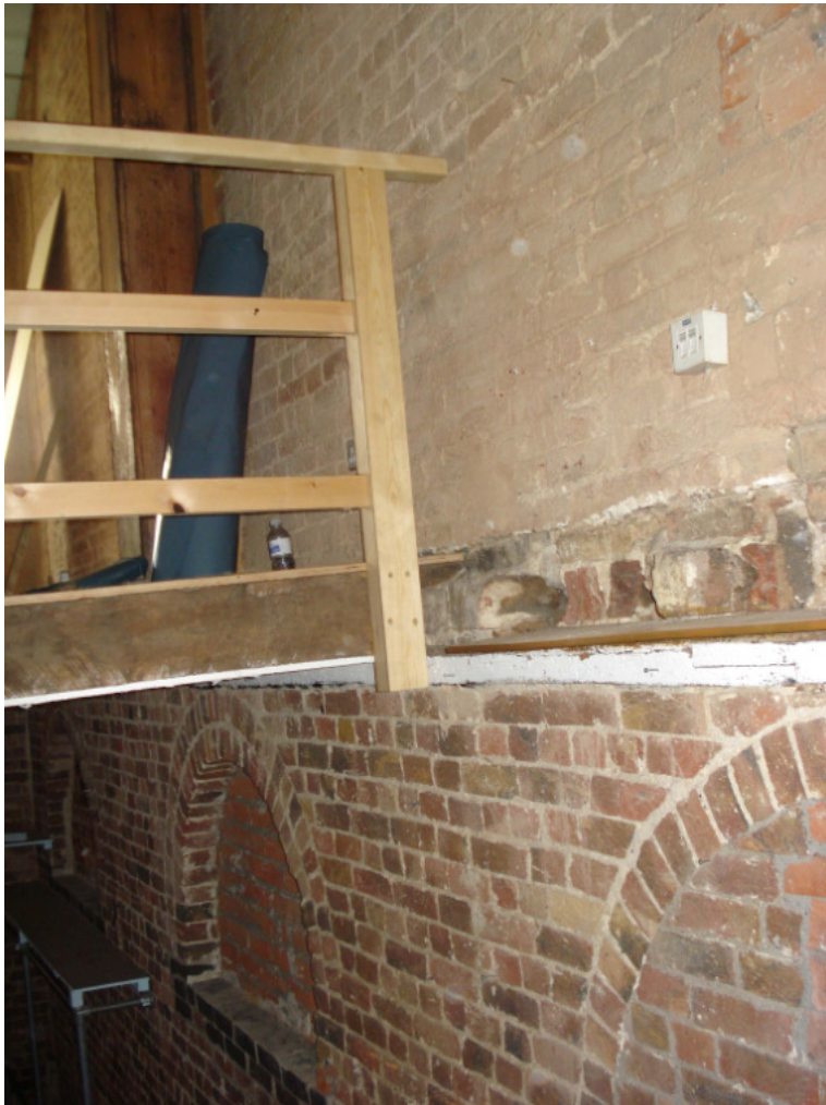
Figure 17: Interior of south elevation pre-demolition showing three infilled arched openings.
