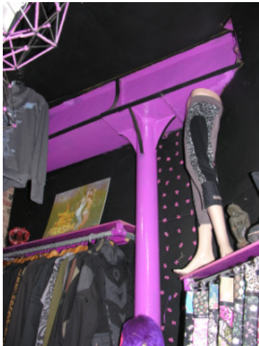
Figure 14: Cast iron column and girder south end interior
