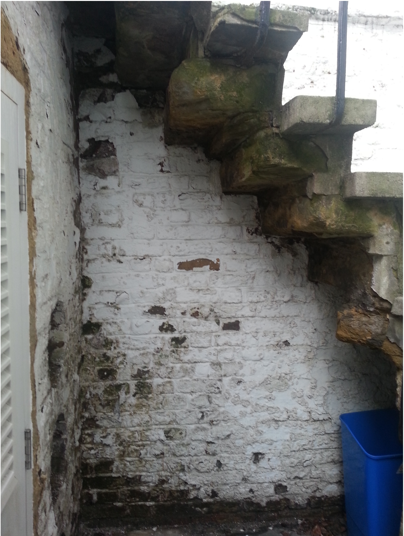
Soffit of showing presumed original stone structure
