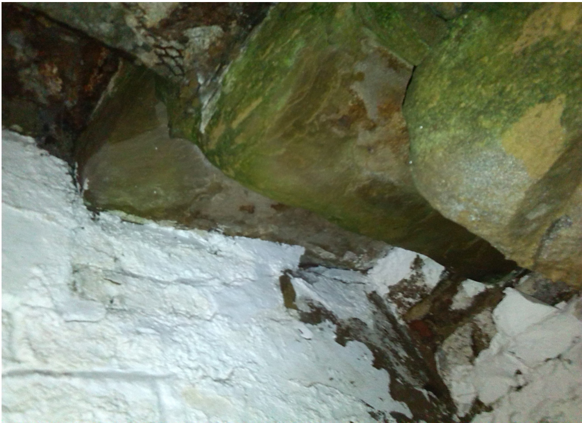
Detail of soffit showing delamination of stone
