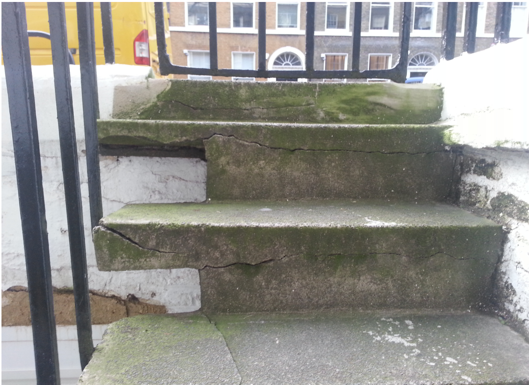
20 th C concrete treads showing spalling and handrail fixings
