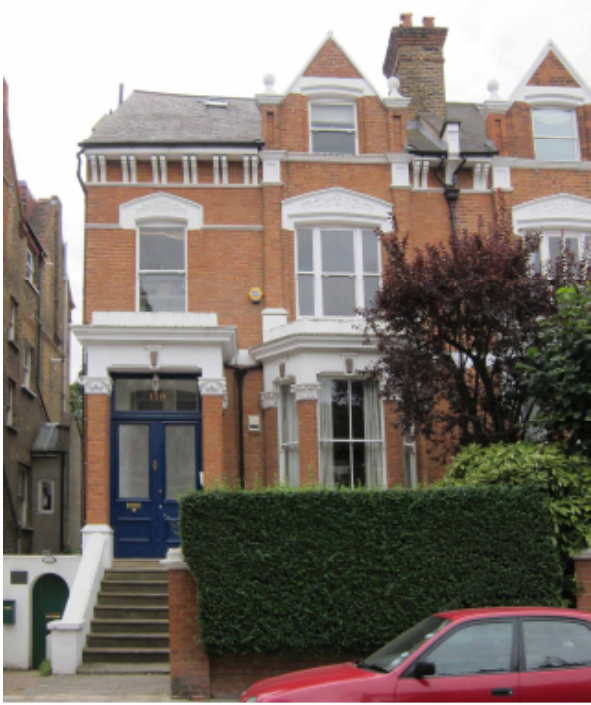
view of front from road ▲
