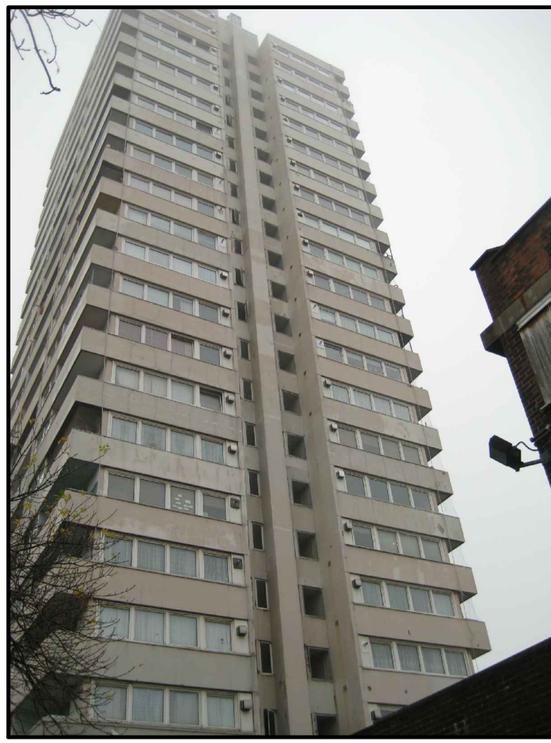
RIGHT HAND SIDE ELEVATION PHOTOGRAPH
