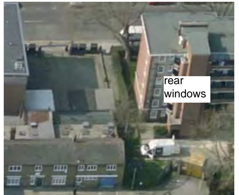
Broomfield House - corner view showing rear windows serving same rooms as side windows
