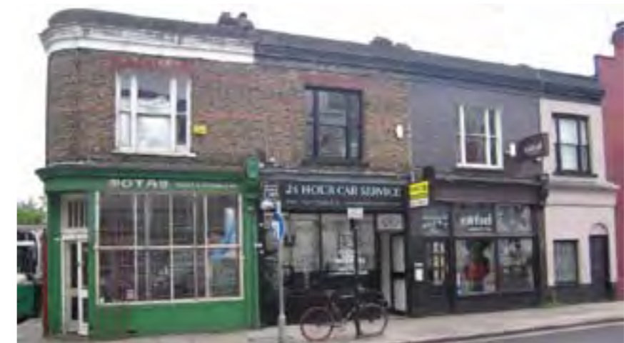
Facade to right of 10 Ferdinand Street
