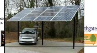
strong structurally roofs due to their heavy weight, especially if the panels are placed on top of existing tiles. The area of PV panels required to generate 1 kWp varies but generally 6-8m<sup>2</sup> for monocrystalline and 10m<sup>2</sup> for polycrystalline panels will generate 1kWp(kWp-energy generated at full sunlight) of electricity.
