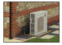
warmer air temperatures. The seasonal efficiencies of air source heat pumps are between 200% - 400%. Heat pumps can operate at outside temperatures down to -15 degC, although there is a drop in COP.
