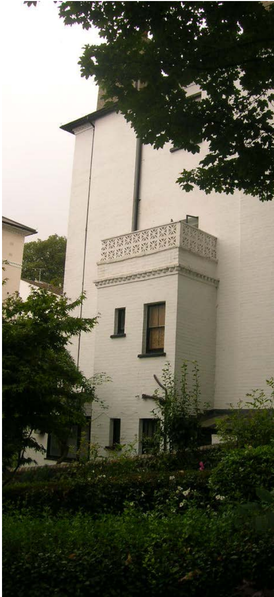
Figure 1 - Photograph taken by Council officer on 8 August 2008.
