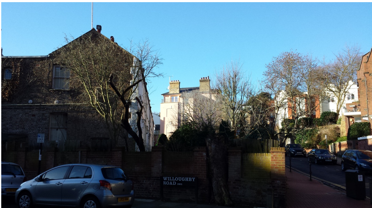
Figure 34 - Photograph taken 29 December 2013 from Willoughby Road, showing Willow Cottages on the left and the rear of 15 Gayton Crescent in the centre of the photograph.
