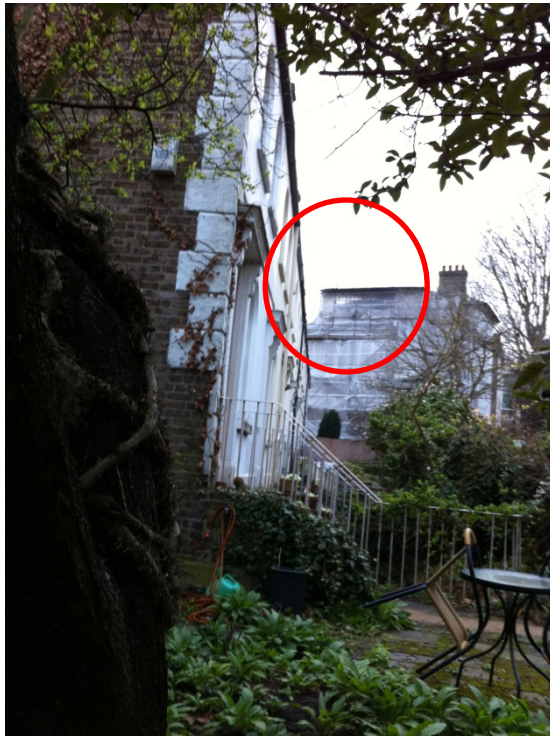
Figure 22 - Photograph taken from Willoughby Road on 28 February 2011 showing southern chimney demolished.
