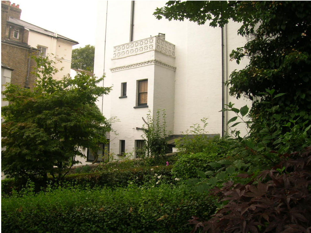
Figure 8 - Photograph taken by Council officer on 8 August 2008.
