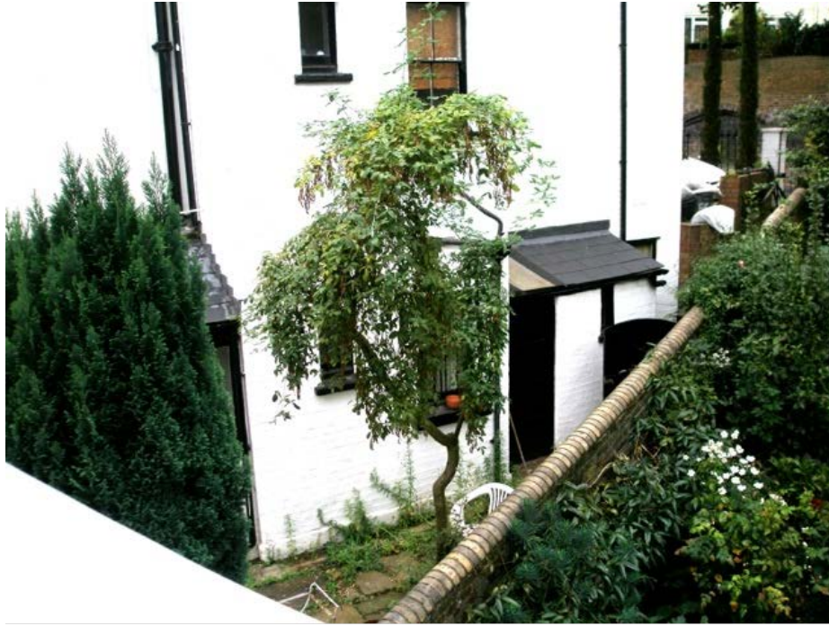
Figure 3 – Dr Swain’s photograph P1011730 of the rear of the property taken between 7 and 13 September 2008 from Willow Cottages showing the two lean-tos either side of the central protrusion. They are simple hut or shed-like structures, subordinate to the main dwelling.
