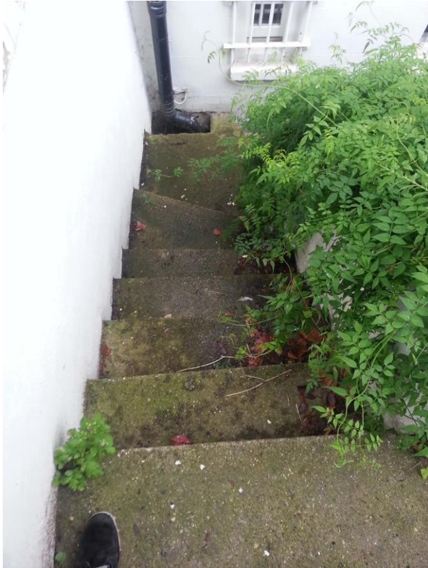
Figure 9: Steps to light well
