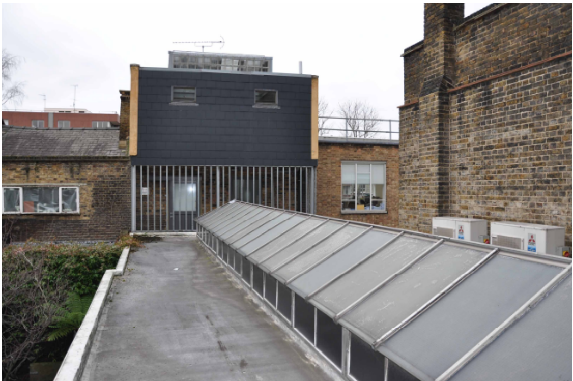
view of existing rear extension roof looking towards No. 11 John's Mews
