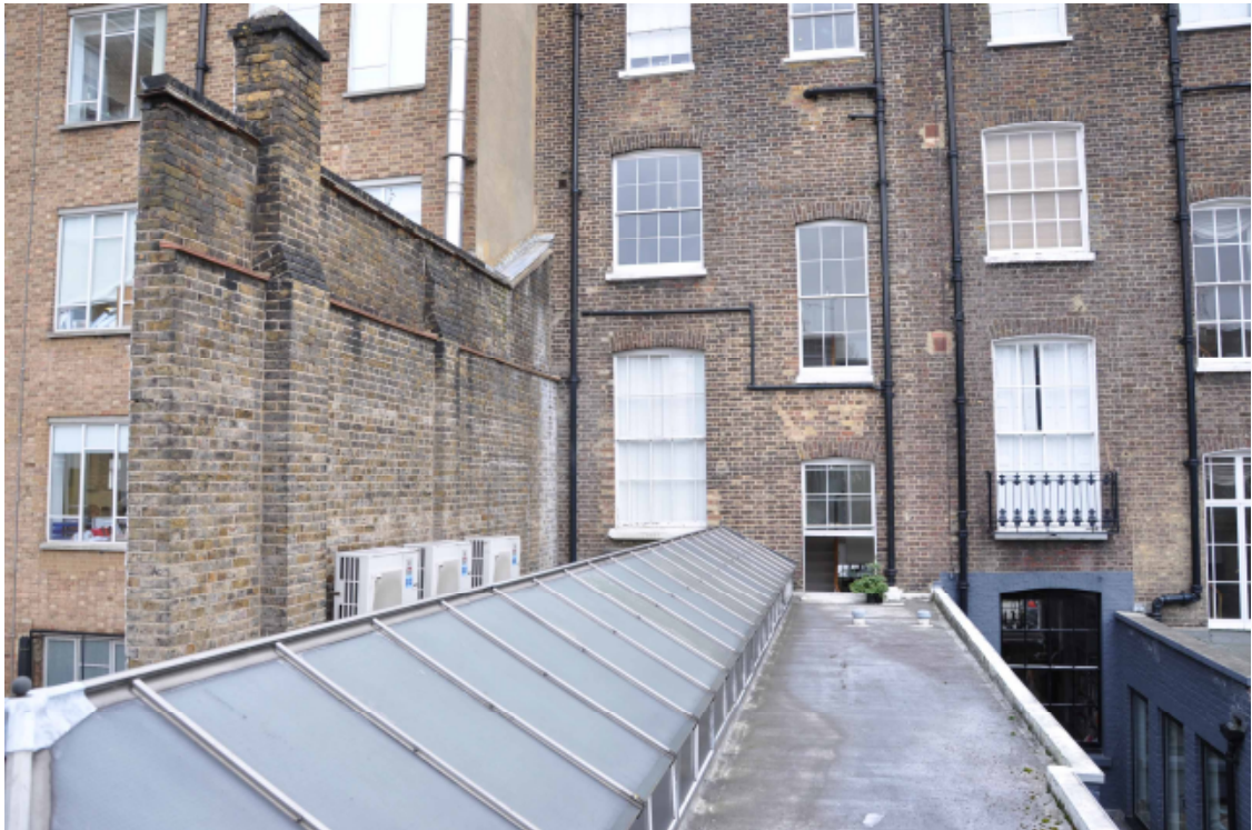
view of existing rear extension roof looking back towards house
