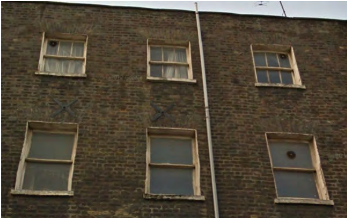
PHOTO 12 - Timber sash windows
