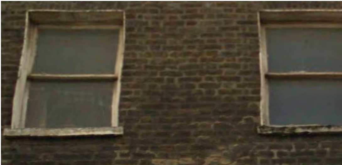
PHOTO 9 - Front view of windows and sub sills in brick wall:
