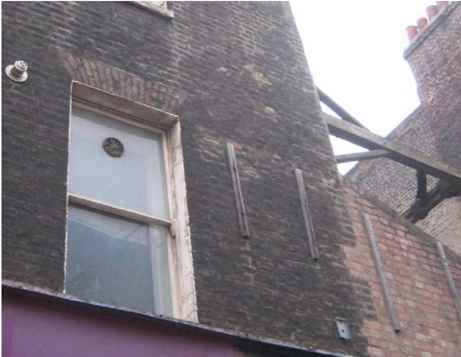
PHOTO 5 - Close up of facade illustrating brick bonding and pointing:
