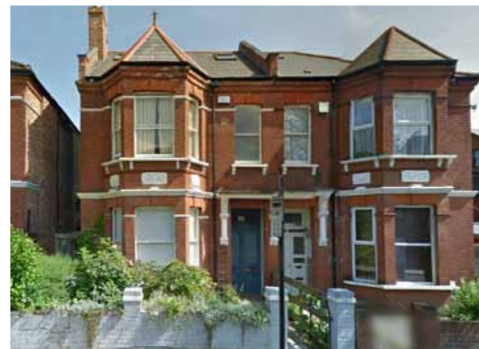
Ebbsfleet Road is typical of the surrounding stock with generous fenestration, expressed entrances and rich detail and texture to the facade
