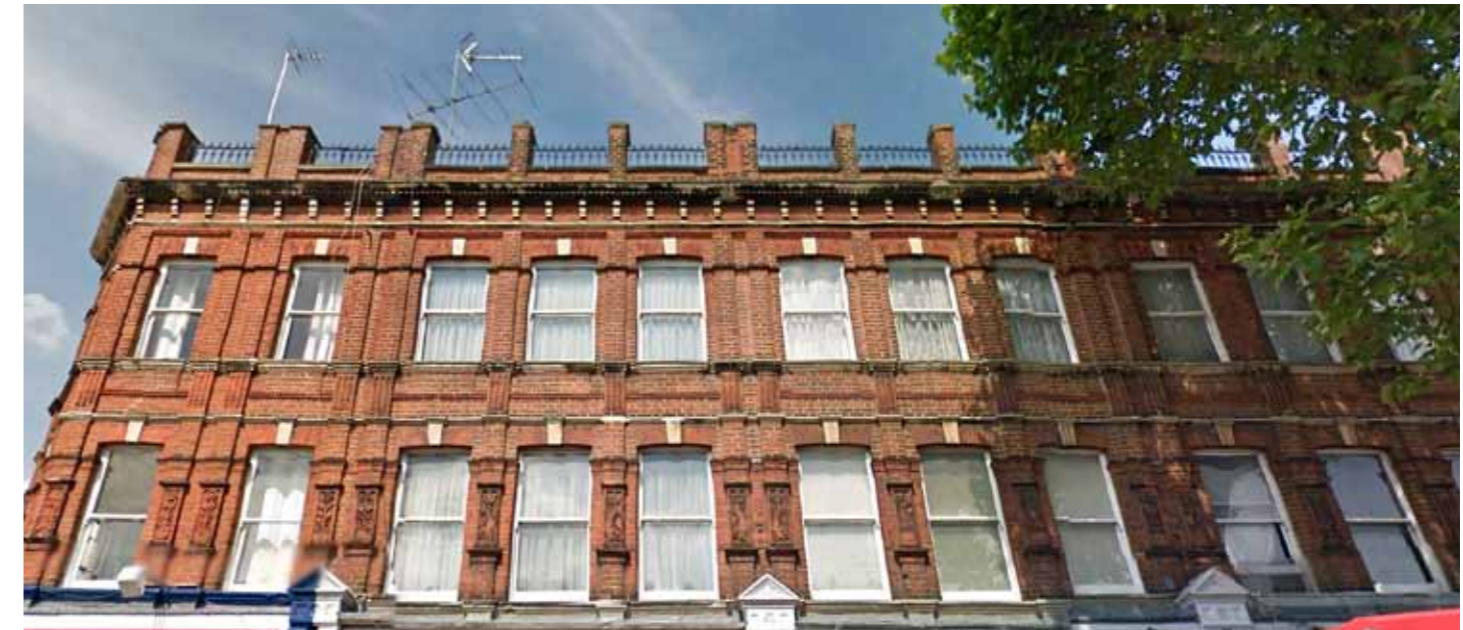
Another more typical example from the high street shows again a strong grided arrangement with games played between horizontal and vertical expressions but with a definite emphasis on the vertical most clearly expressed by the windows
