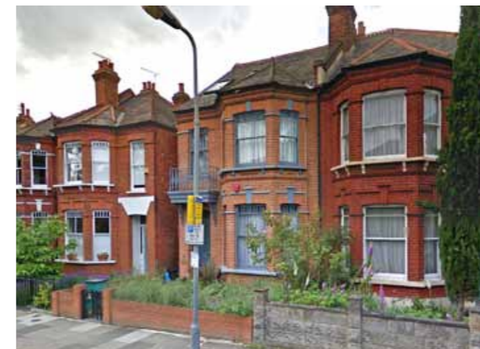
As shown by this photo from Richborough Road the red brick stock, mortar and detailing all vary
