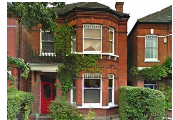
The bay windows dominate the facade with larger areas of brick work broken down by banding and other brick detailing
