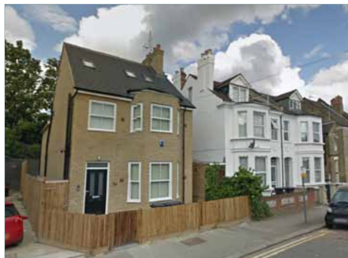
Two storey buildings on Oak Grove, where the roof space has been converted into a third storey
