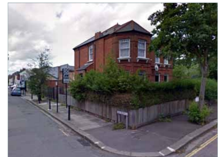
19 Richborough, a two storey red-brick Victorian detached building with a pitched roof, with its main elevation towards the south onto Richborough Road
