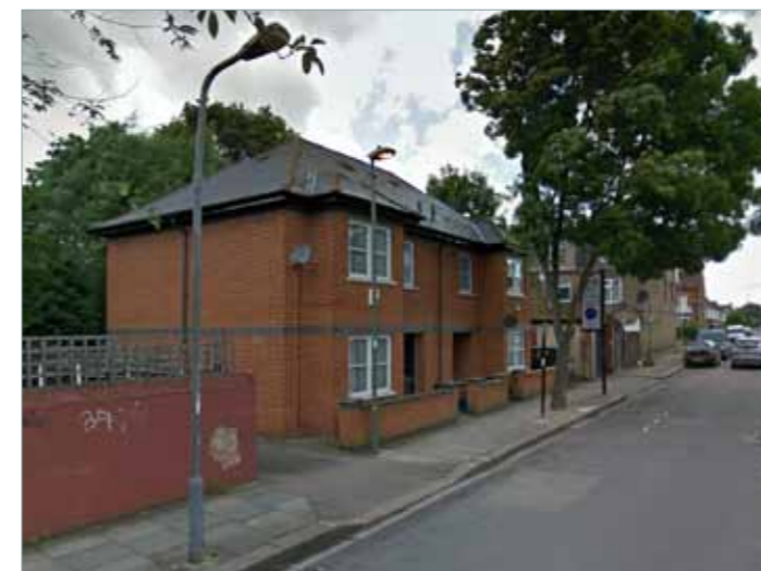
A more recent built, 58-60 Oak Grove - opposite the site - is a semi-detached red-brick building with grey soldier courses at ceiling level and white windows
