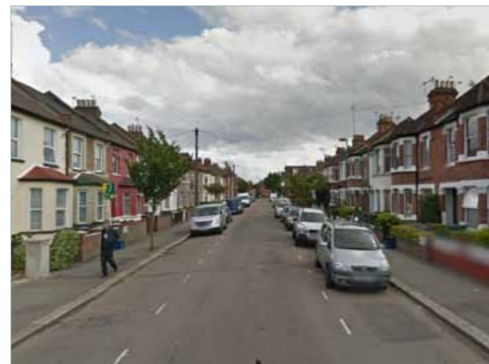
Oak Grove (looking south) consists of terraces of two storey Victorian houses with pitched roofs, brick or rendered facades and bay windows
