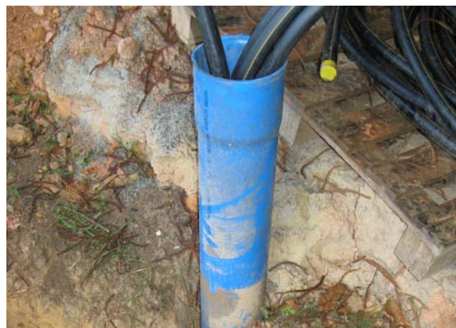
Example of GSHP borehole pipework.
