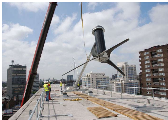
A building-mounted 6kW Proven wind turbine
