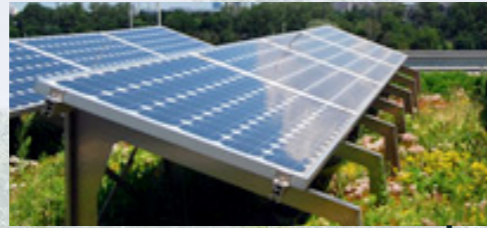
PV. panels layed on greenroof
