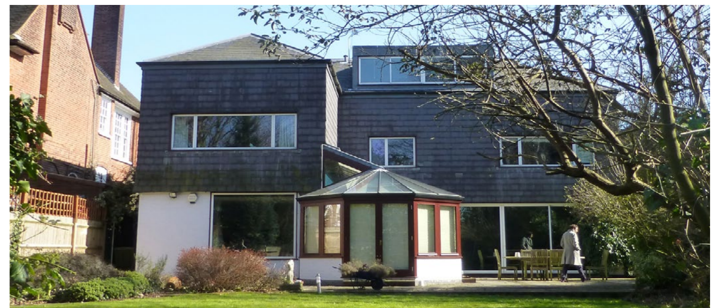
Existing Residence: Rear
