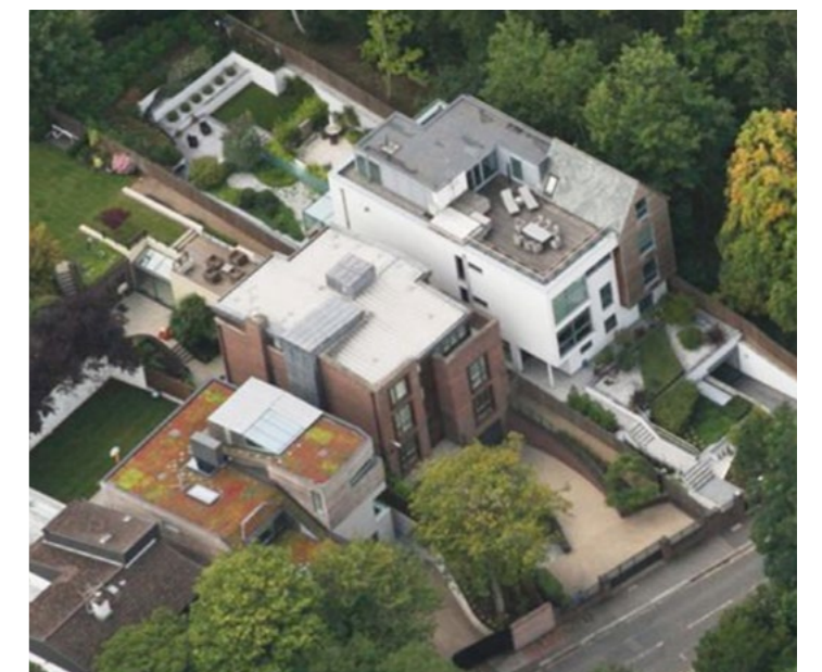
Roof terrace along West Heath Road
