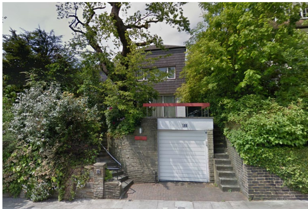
View of the site from the second crossover.
