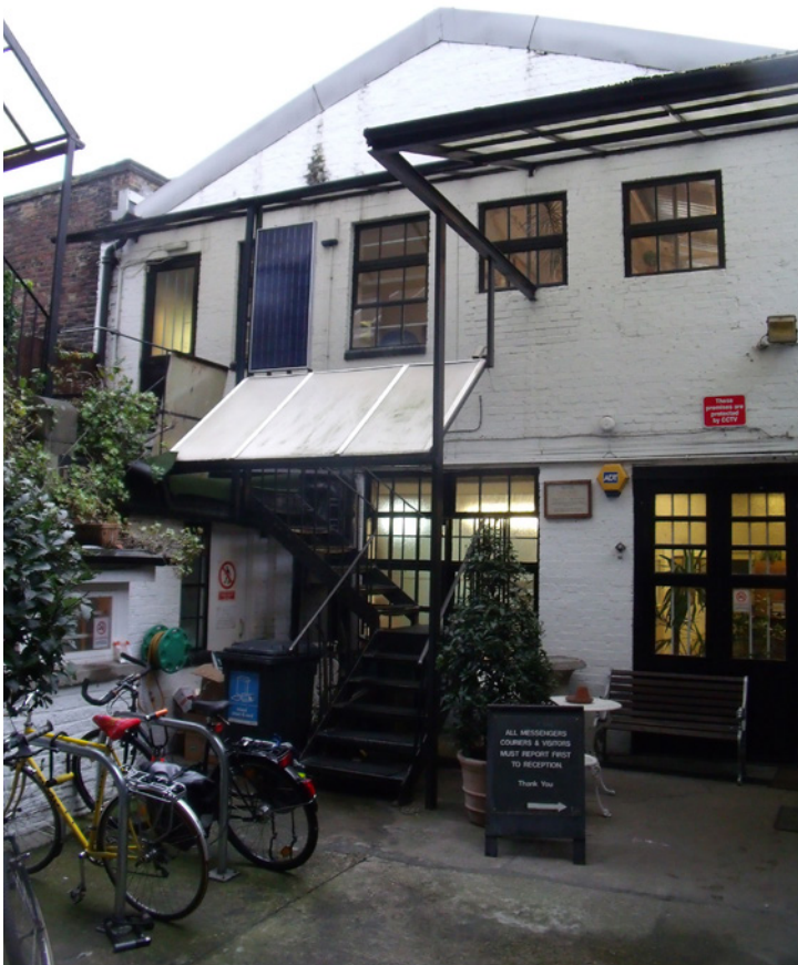
3. View of the front of the industrial infill building at the rear of the site, viewed from the courtyard
