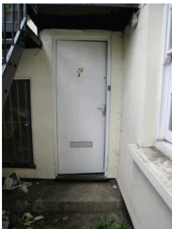
basement flat entrance
