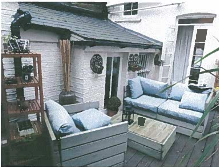
Photograph of existing first floor extension.
