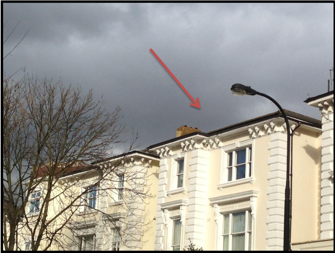
View to roof from street
