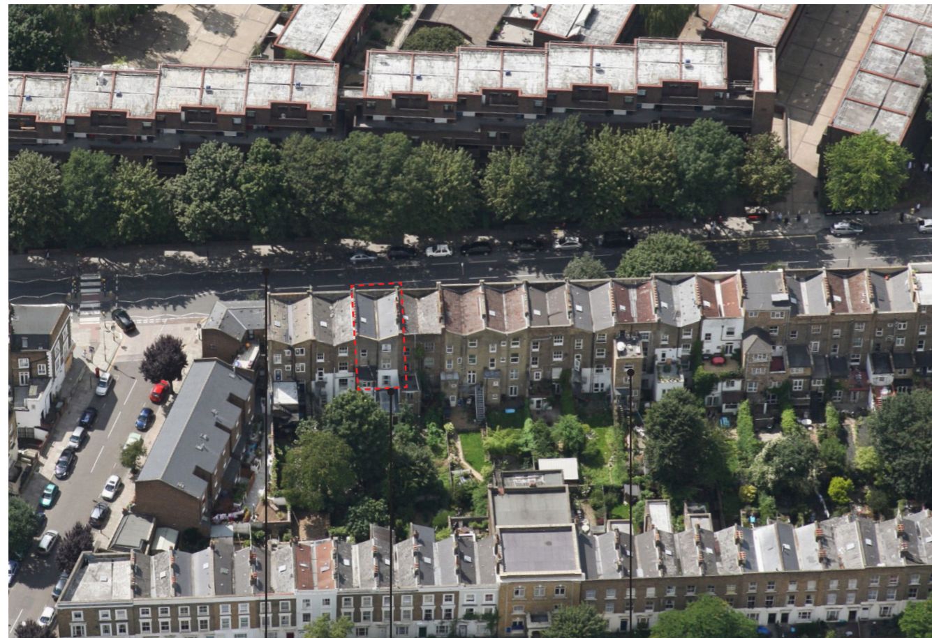
FIG 5.1 Frontage of the site and adjacent properties.
