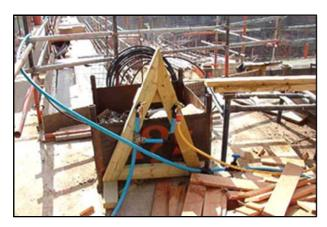
Example opposite of a temporary watering system hub rigged up on site to provide adequate mains watering feeds to different roof areas.
