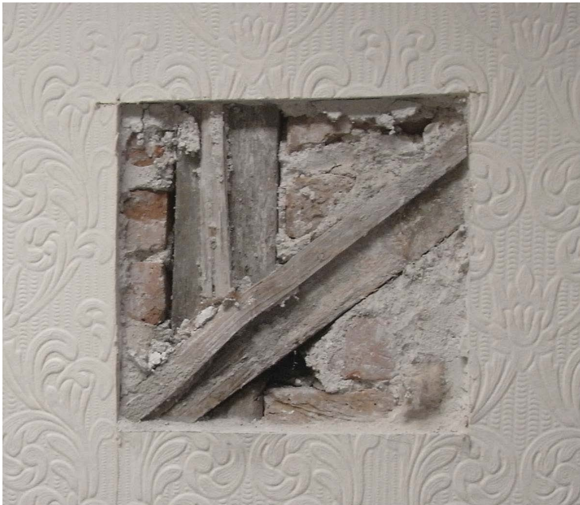
Photograph 2: Masonry infill to timber framed wall, entrance hallway to Ground Floor of No. 46 (see 3.2.1 within report).
