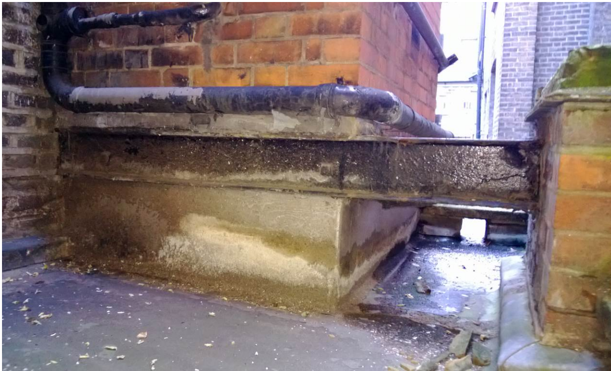
Photograph 5: Steel beam supporting side extension (see 3.6.1 within report).
