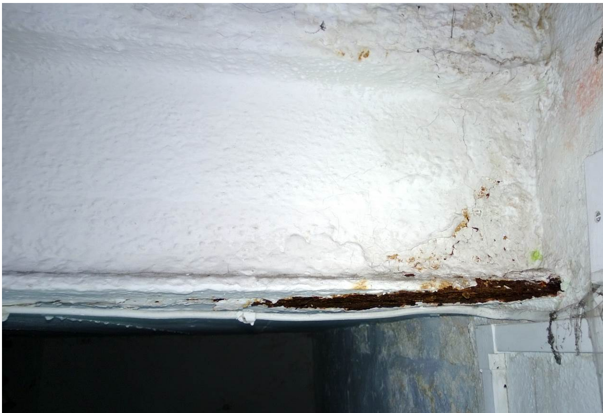
Photograph 6: Corroded external steel beam to rear of No. 47 (see 3.1.6 within report).
