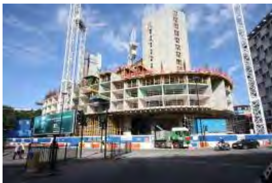
Westminster Park Plaza, London Construction of new luxury hotel by top-down method incorporating 4 basement levels
