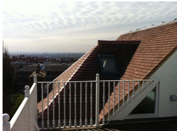
(4) Photo of the existing roof from Terrace.
