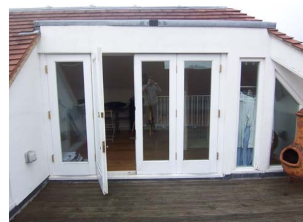
(10) Photo of the existing terrace doors
