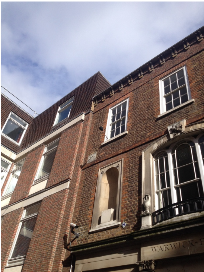
Measurement on the front façade of the development
