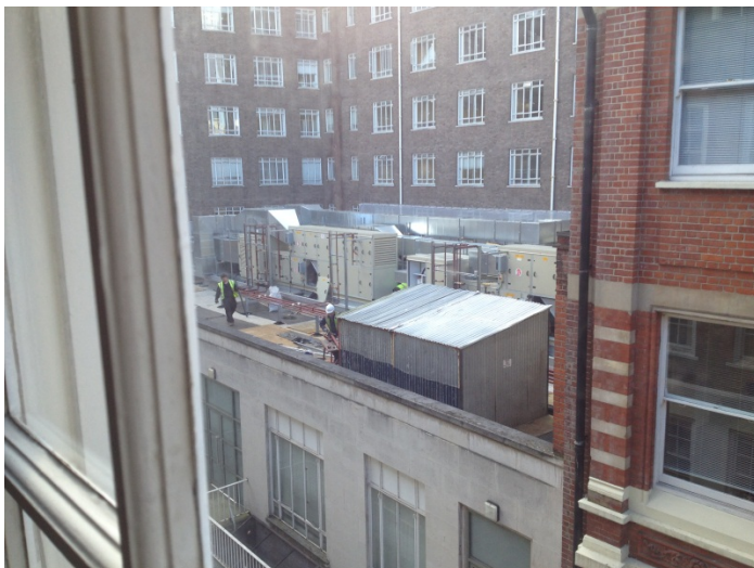
View of Plant from the “Warwick Street” façade.
