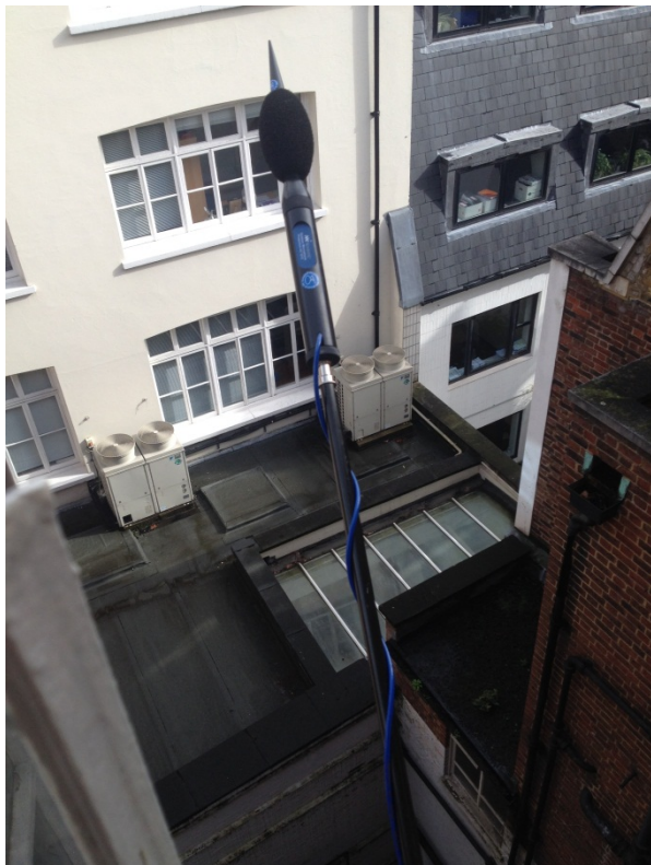
Measurement on the rear façade of the development
