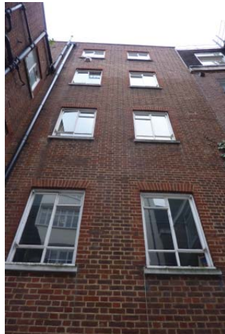
8 Warwick Court Rear elevation as viewed from lightwell
