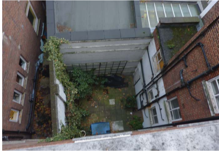
8 Warwick Court Rear lightwell as viewed from high level window
