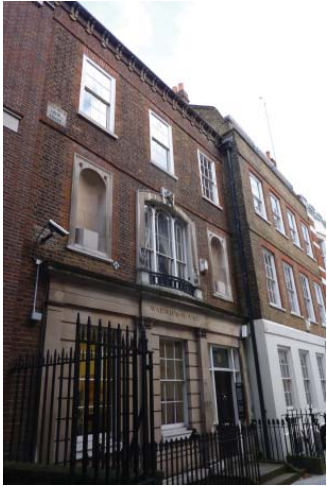
8 Warwick Court Street view looking South
