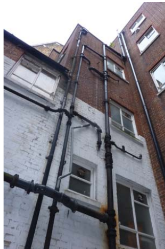
8 Warwick Court Closest wing extension as viewed from lightwell
