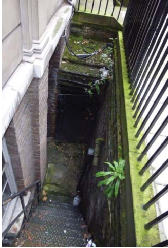
8 Warwick Court Front Lightwell
