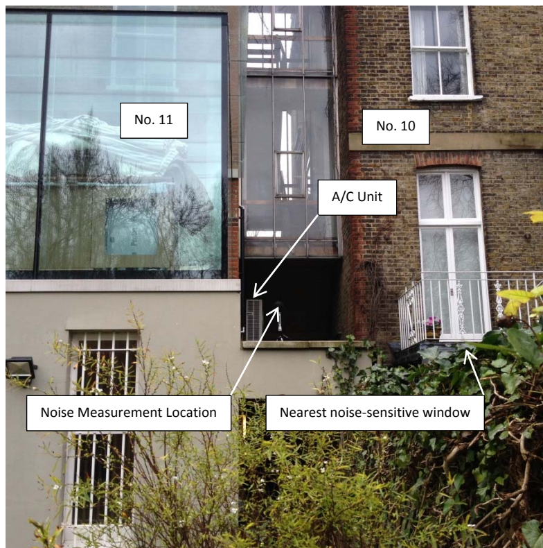
Photo 1. South East (Rear) Elevation
