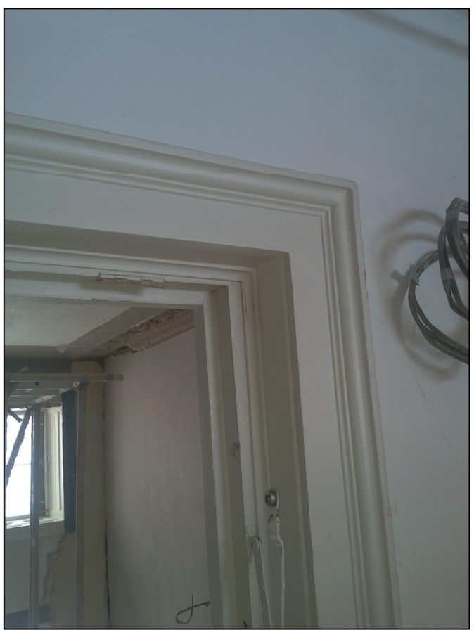
existing architrave from first floor
