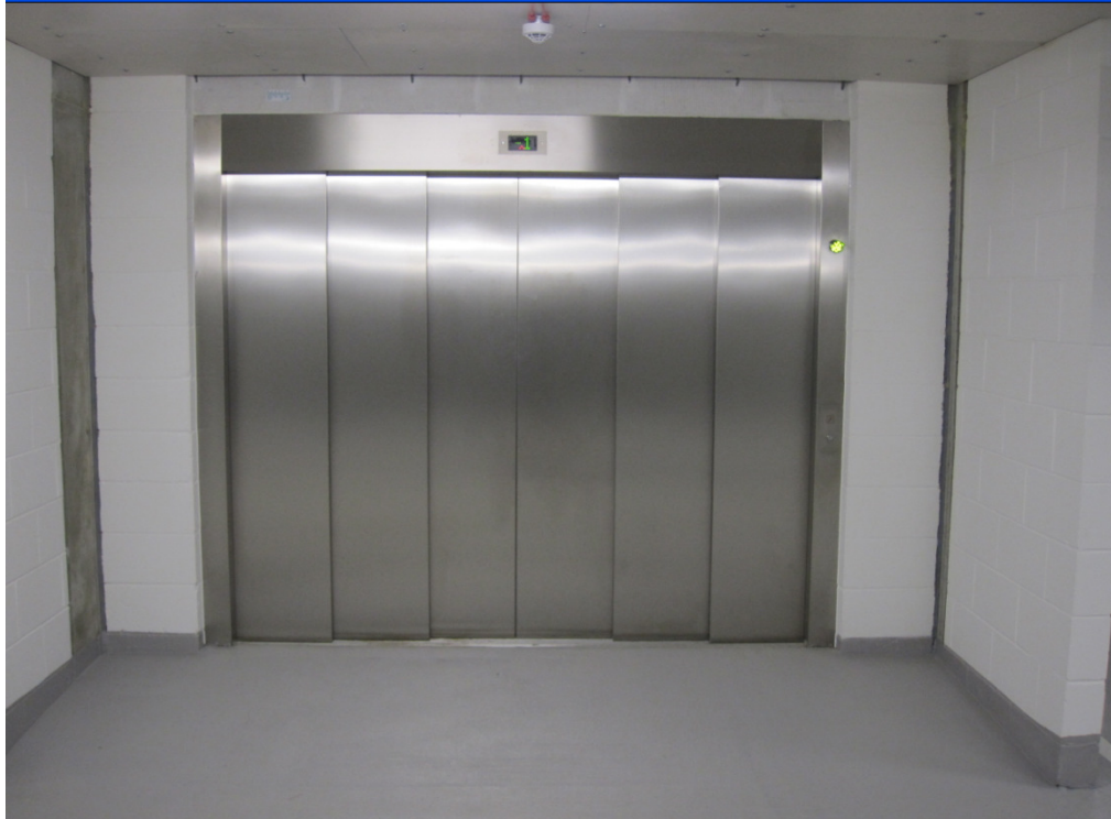
Fig 1 – Photograph to show the proposed design of car lift entrance doors. Doors are to be constructed from steel and powder coated in RAL 7038 (not finished in stainless steel as shown in this photo).
