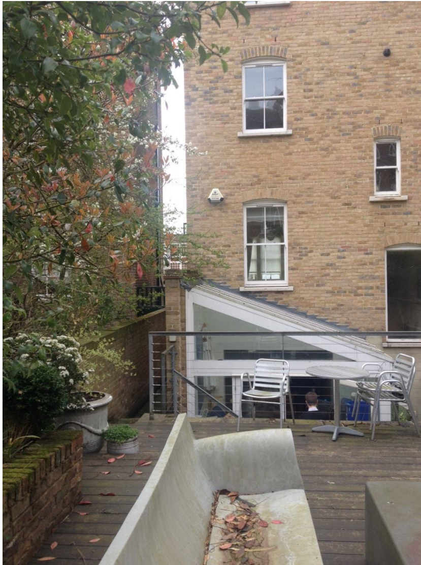
Photo 2- Looking toward existing rear extension, window on right hand side to become door
