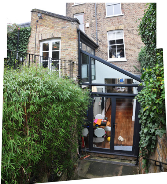
view of existing rear closet wing and glazed extension (no works to this elevation)
