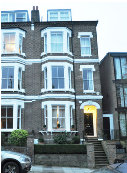
view of front facade
