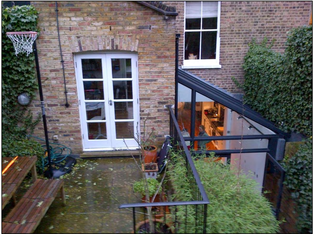
Photograph Three: Rear garden in No. 33, showing the variable ground levels.
