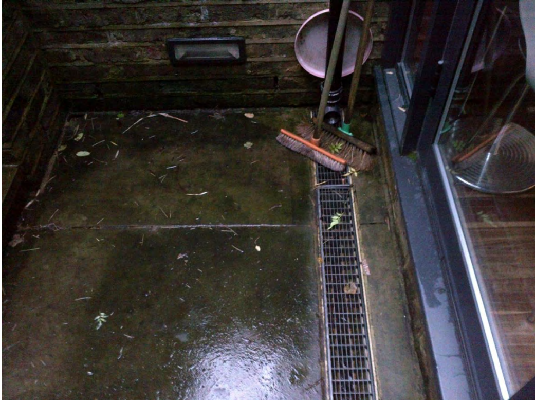
Photograph Five: Channel drain in rear garden patio area.
