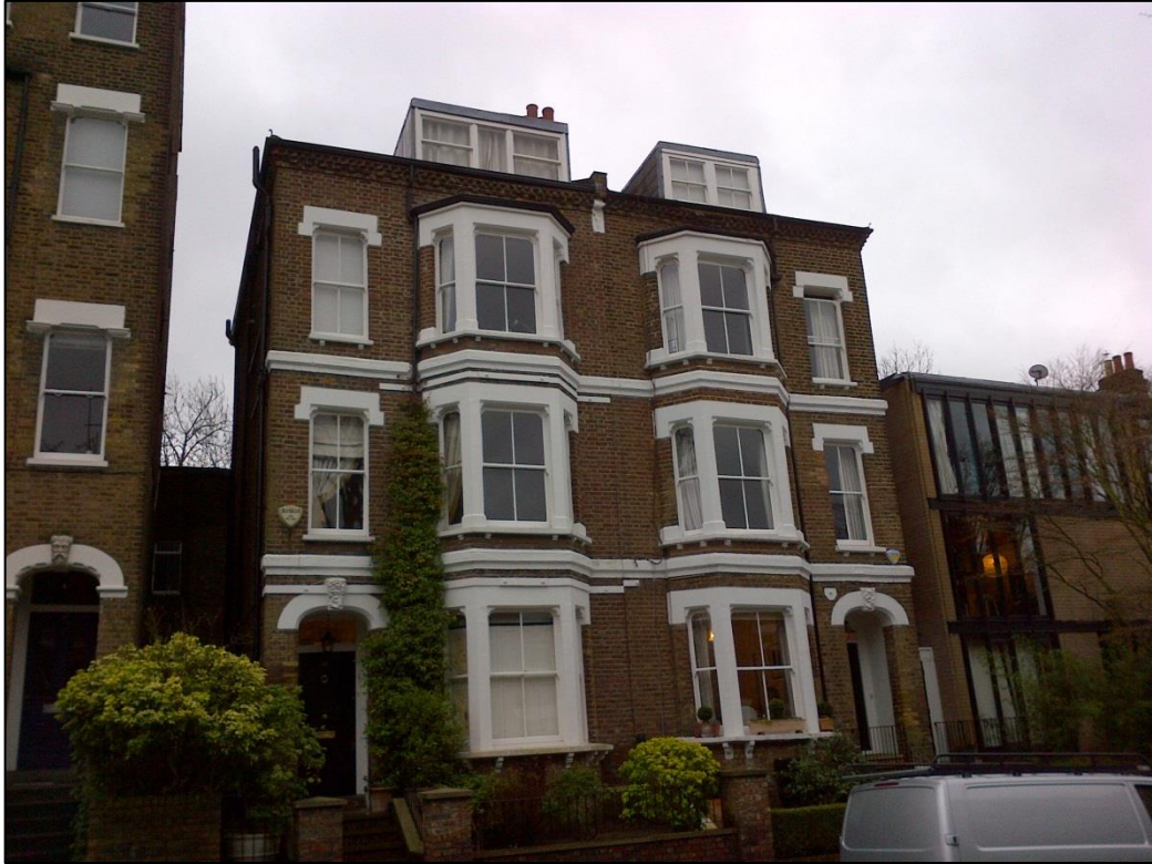
Photograph One: Front view of 35 and 33 South Hill Park. Note the strapping above and below bay windows of No. 35. No. 33 has had them mostly removed, but wall bolts still remain visible.
