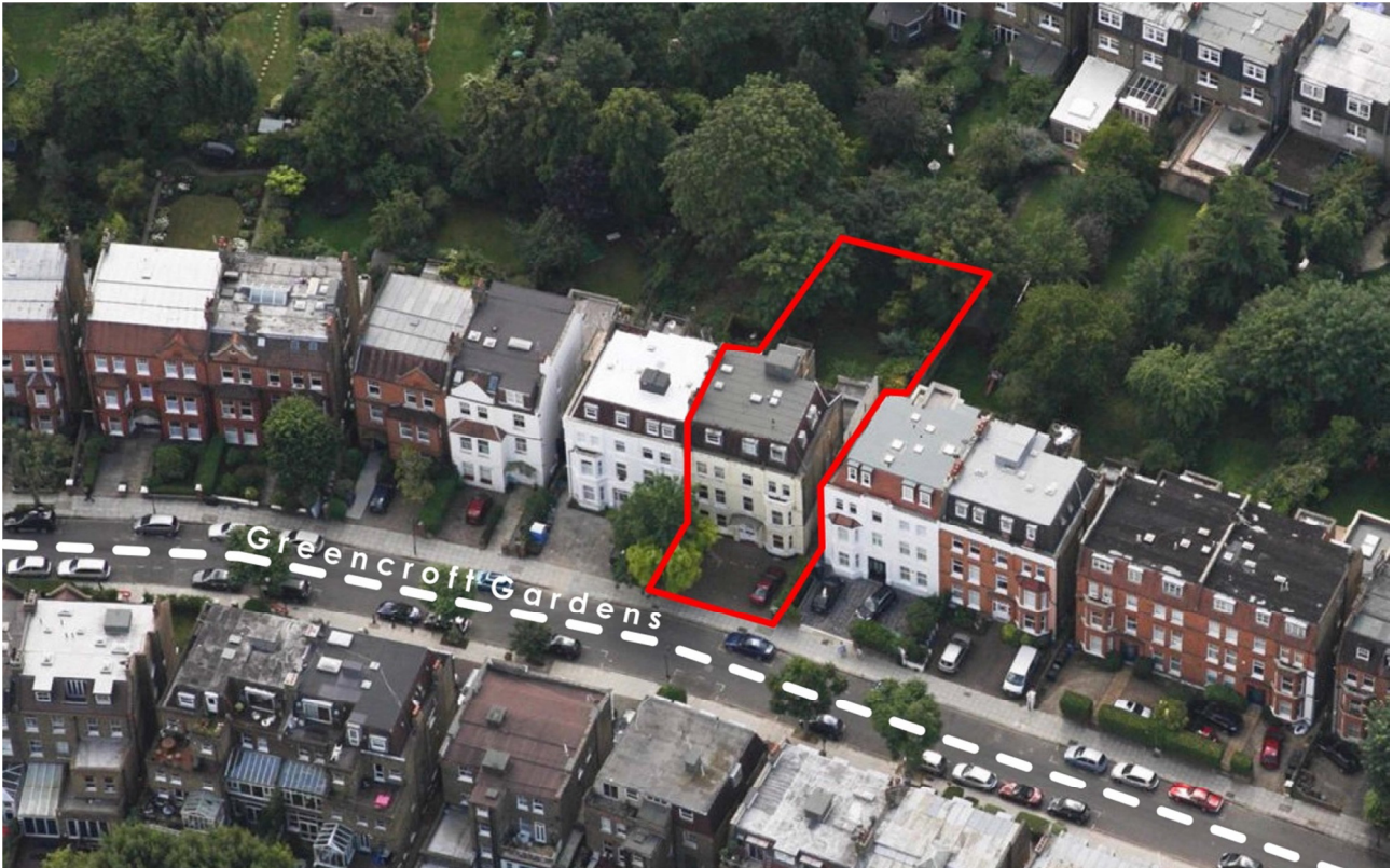
Fig. 1; Aerial View of No. 85 Greencroft Gardens, London NW6 3LJ (property outlined in red)
