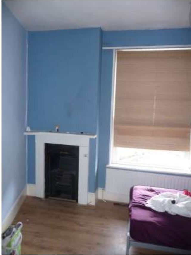
Second Floor fireplace to be retained.
