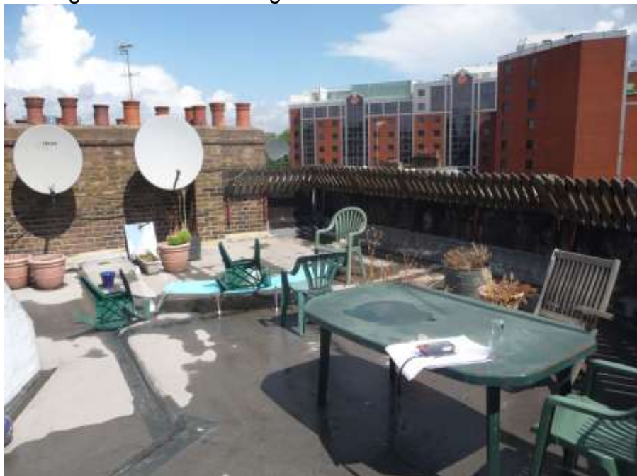
Existing roof terrace looking north
