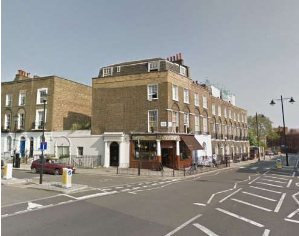
Junction of Amwell Street and River Street
