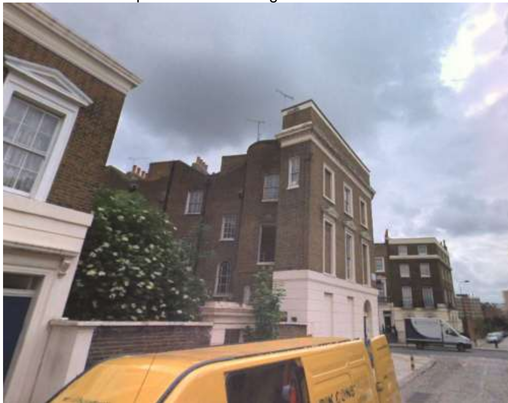
Junction of Calthorpe Street and Gough Street
