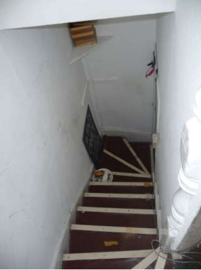
Ground to First Floor staircase to be removed and replaced.
