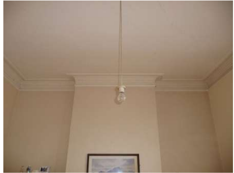
First Floor cornice to be retained and preserved.
