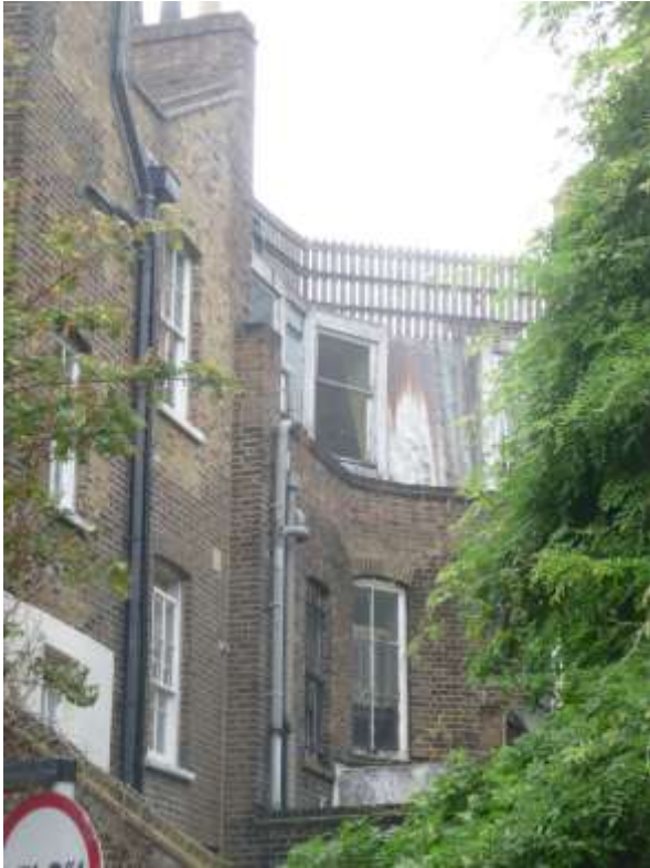
View from Wren Street showing existing mansard roof.
