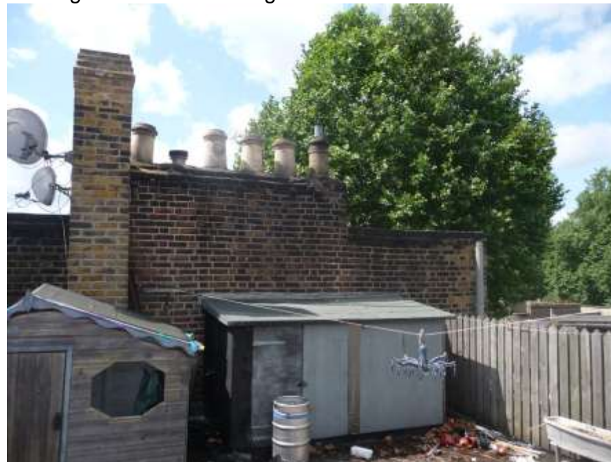
Existing roof terrace looking south
