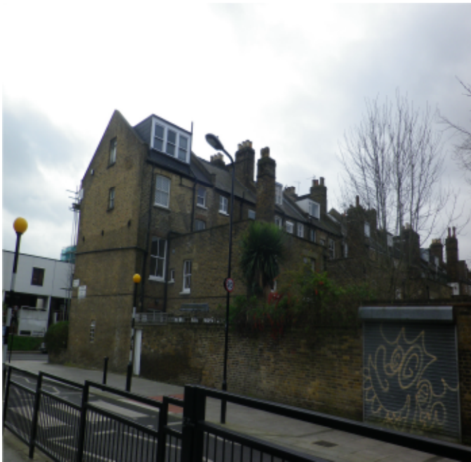
Photo 1 – The rear of properties along Mansfield Road
