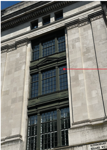
Reinstated glazing in existing window frames (External Bloomsbury Square)
