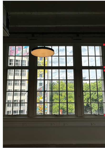
Reinstated glazing in existing window frames (upper 2 panes). Limited amounts of existing glazing were located on site and where possible these were used in the re-glazing exercise. Frames redecorated
