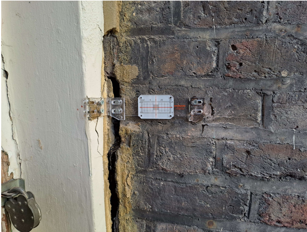
Photograph 1: tell tale monitor installed across junction
