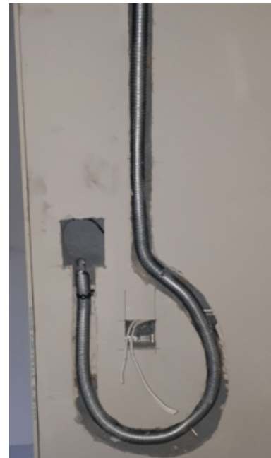
EXAMPLE WALL CHASING 40X40MM FOR AUTOMIST HOSE
