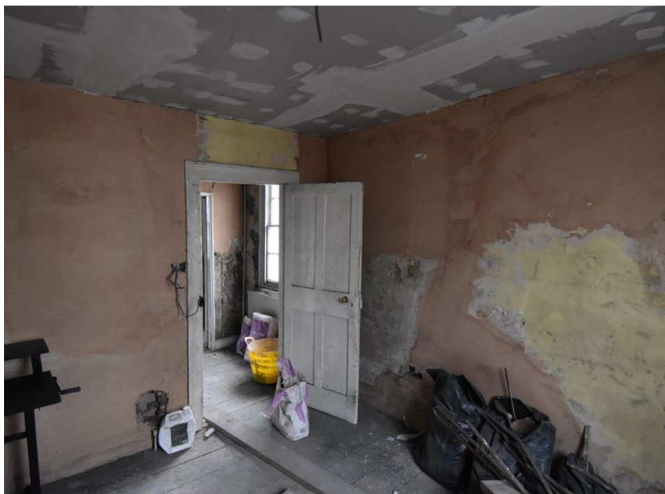
3.17 F1 front bedroom showing recent ceiling and patched plasterwork
