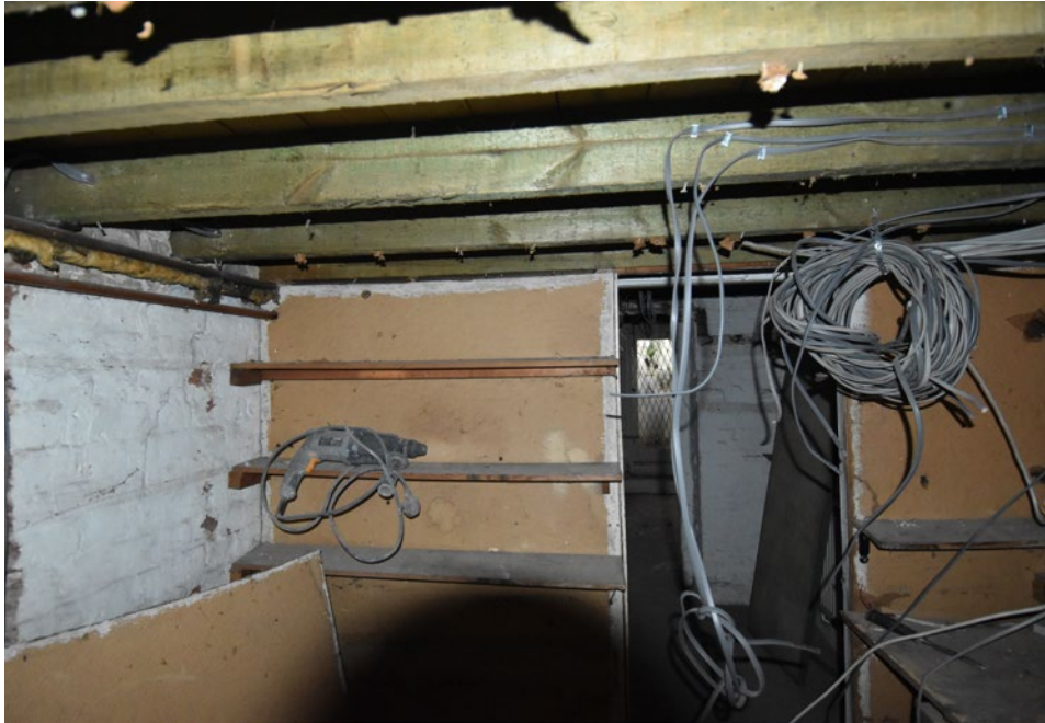
3.10 B4 showing modern joists and modern partition wall
