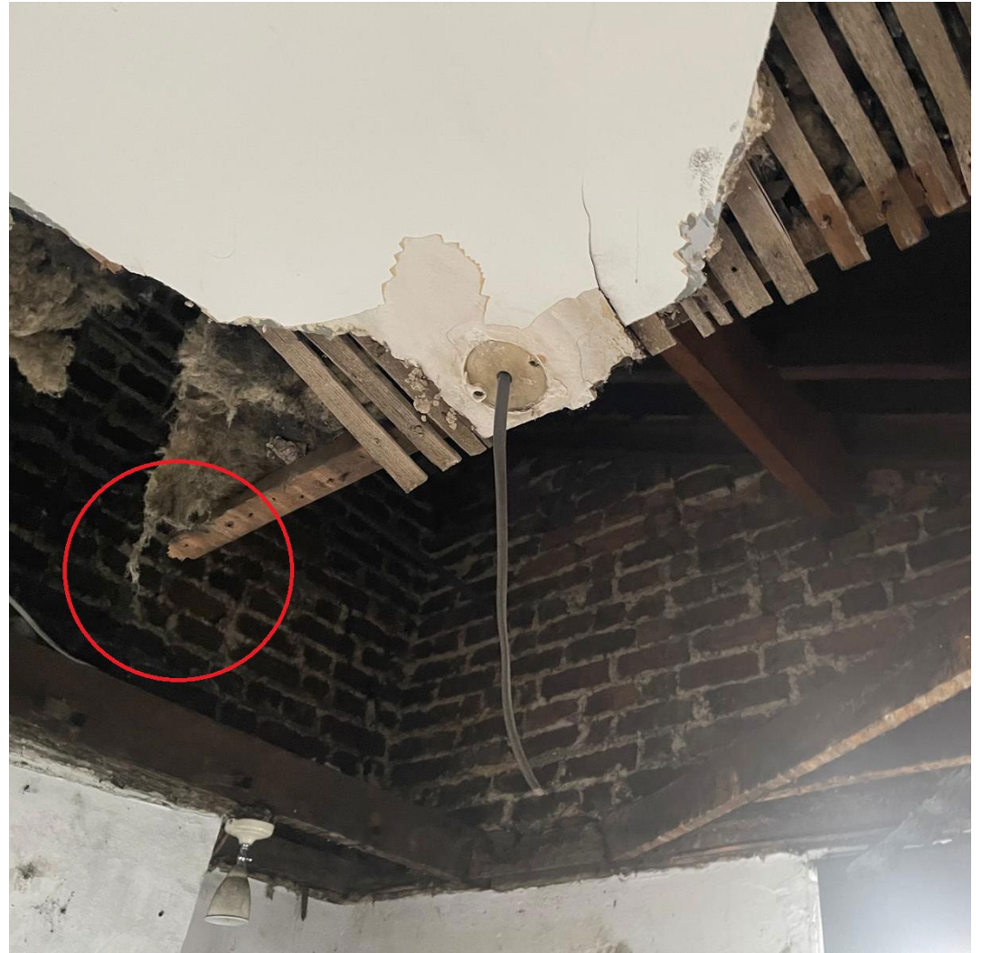
3.20 Ceiling in F2 during works showing failure of joists
