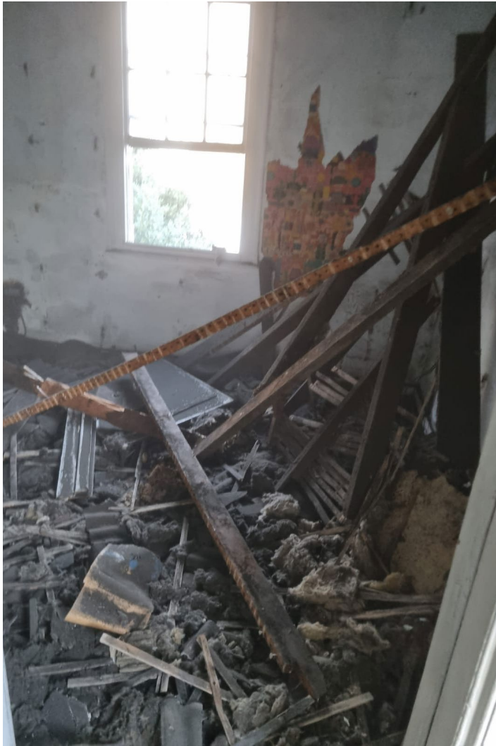
3.21 Room F2 after the ceiling collapse
