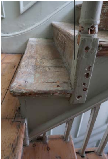
I.1 newel post was moved up one step and cut in and screwed to stringer.
