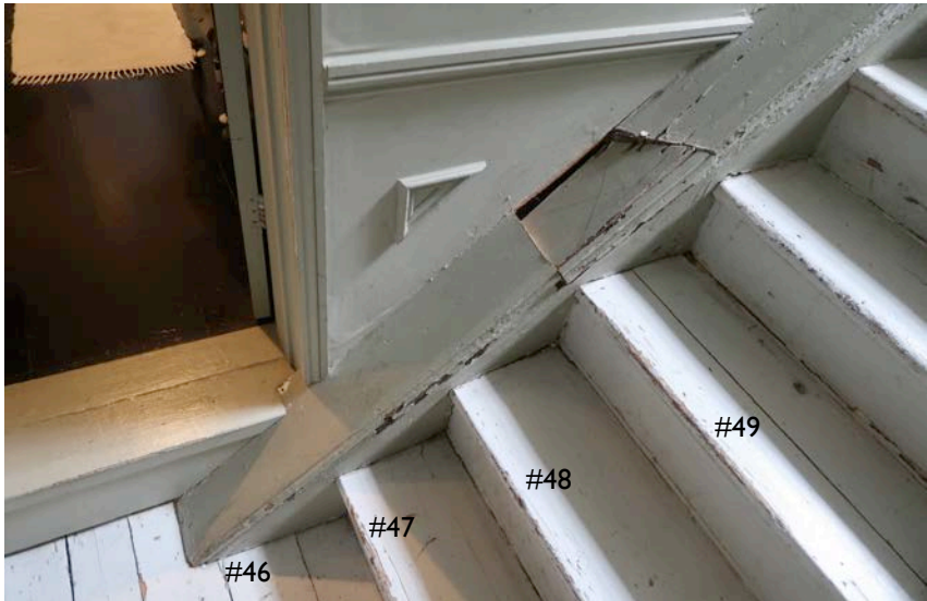
When the third floor infill partition was rebuilt to enclose under the third to fourth floor flight it was positioned out in the stair well. This caused a hazard of head and shoulder collision and so the lower flight was boxed in along the side which reduced the stair clear width. The landing outside the bathroom and the first three treads of the flight up are later alterations to this flight which was first built as a dog-leg.
