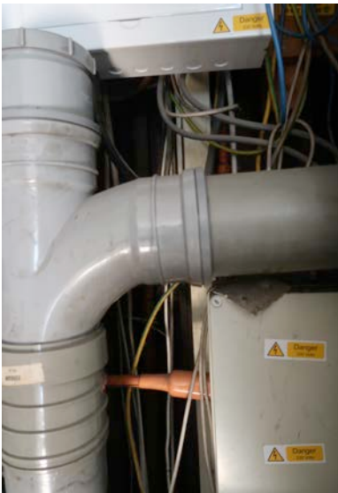
I.2 riser congested with water, gas, electrical and foul wastes services plus redundant services without support, containment or fire compartmentation or fire barriers, in shaft of former goods hoist up from ground floor retail.
