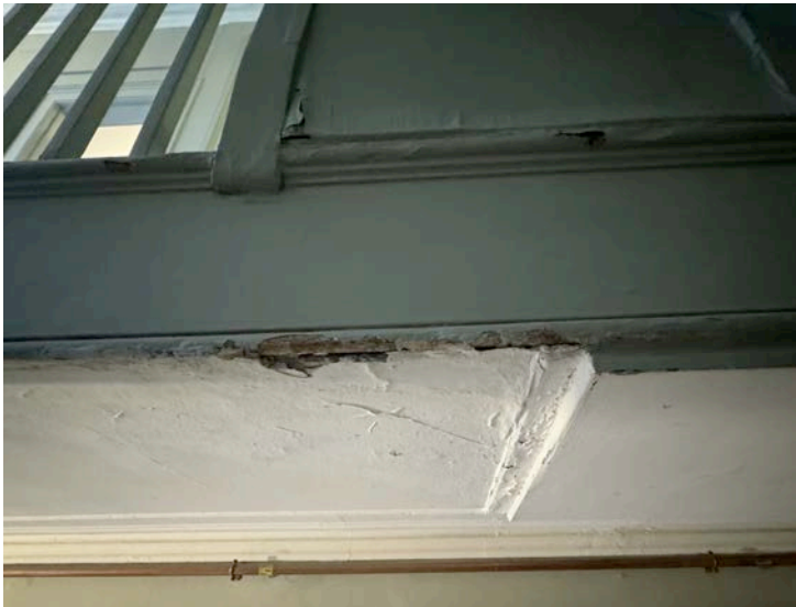
Looking up from below at NEWEL 2B, installed in 1976 which was cut into the side of the second floor fascia through the 1848 edge moulding. The soffit to the right has been underlined with boarding and a crude plaster band added. NEWELS 2A and 2B appear to be reused square posts with chamfers and NEWEL 2B was cut to a taper on the back. There is a hardboard infill between the newels at low level.
