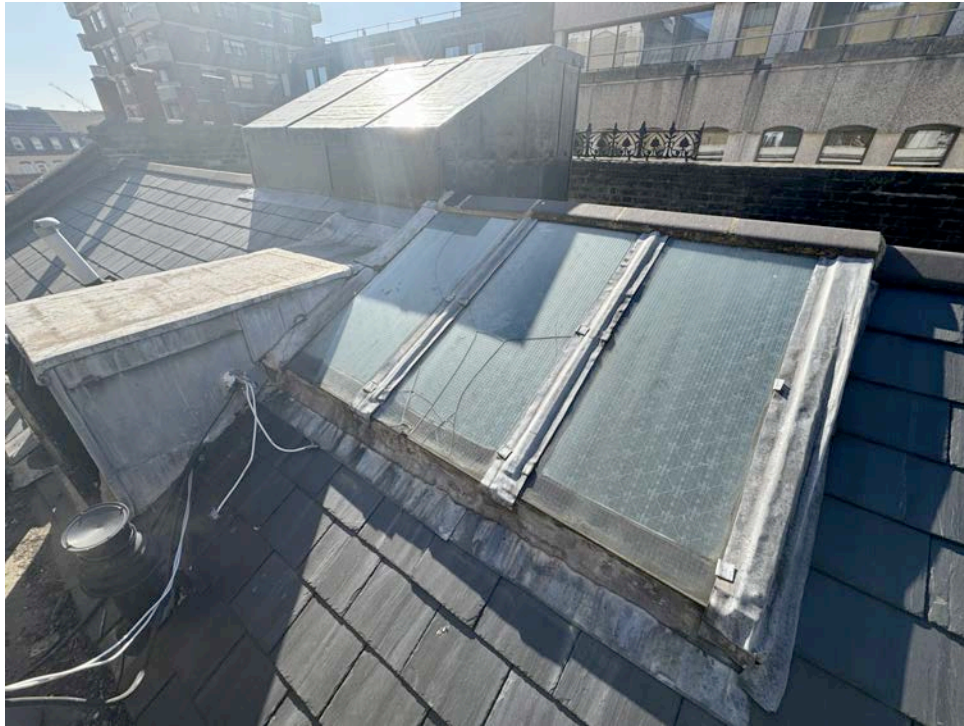
Rear slope of roof with roof access overrun enclosure on Newton Street face and surviving half of rooflight on rear face.
