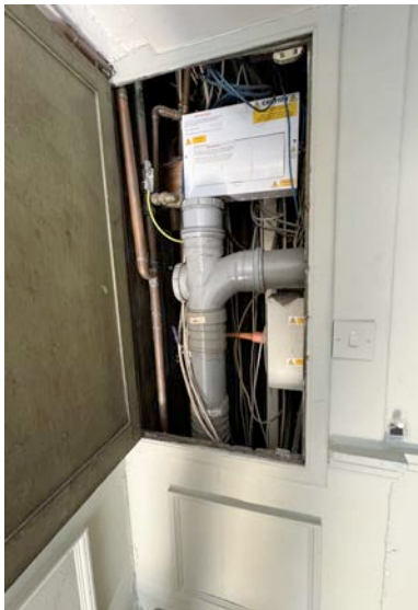
I.2 riser congested with water, gas, electrical and foul wastes services plus redundant services without support, containment or fire compartmentation or fire barriers, in shaft of former goods hoist up from ground floor retail.
