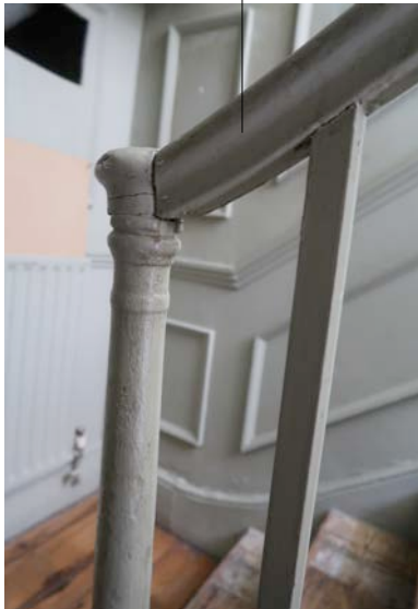
I.1 newel post was moved up one step and cut in and screwed to stringer.
