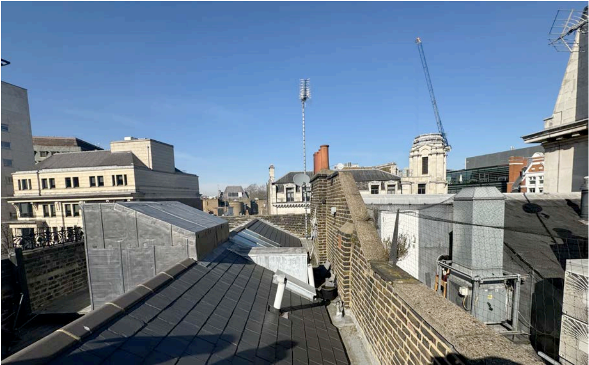
Rear slope of roof with roof access overrun, surviving half of rooflight on rear face and modern hatches across the ridge line.
