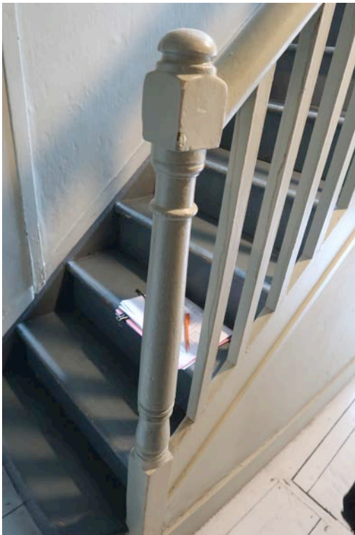
Relatively modern treads with less wear than flight below and turned newel post apparently re-used from first construction of this flight, matching newel at top of stair. Newel and stair sit on the floor, not built into it. Fibre board infill above stringer (far) and hardboard infill below stringer (near).
