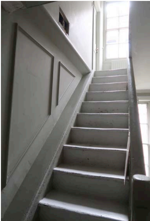
Looking up from below at NEWEL 2B, installed in 1976 which was cut into the side of the second floor fascia through the 1848 edge moulding. The soffit to the right has been underlined with boarding and a crude plaster band added. NEWELS 2A and 2B appear to be reused square posts with chamfers and NEWEL 2B was cut to a taper on the back. There is a hardboard infill between the newels at low level.
