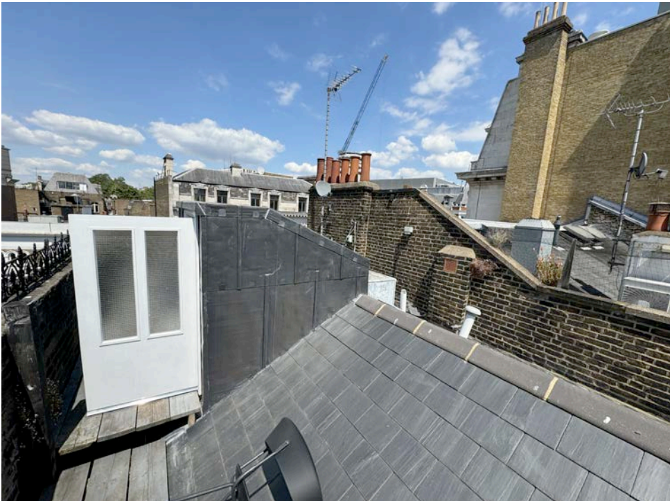
Newton Street front slope with roof access overrun and deck on steel frame to lesser width than permitted in 2008. Victorian style crested parapet is apparently modern.
