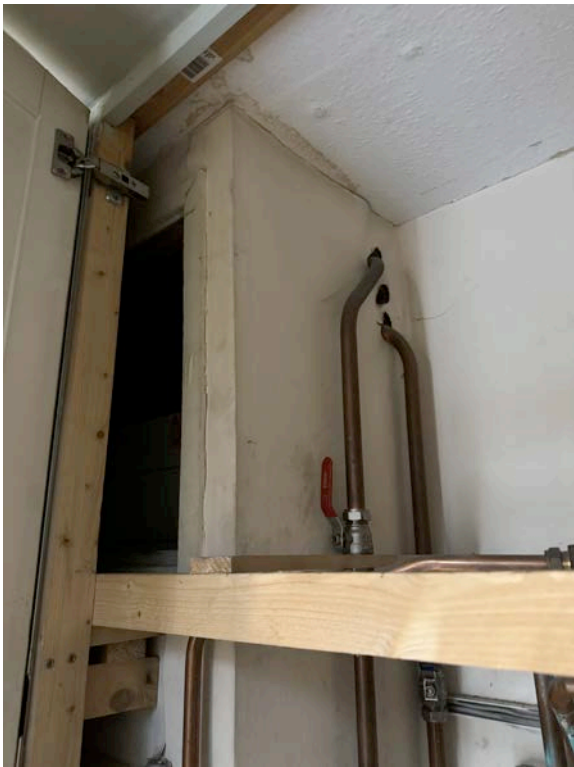
3.7 riser within hot water cylinder cupboard. Riser congested with water, gas, electrical and foul wastes services plus redundant services without support, containment or fire compartmentation or fire barriers.
