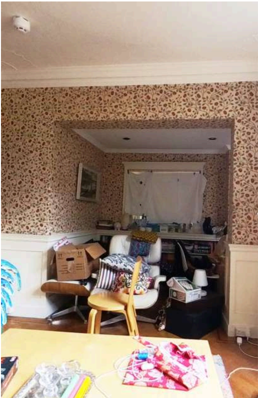
Ground Floor Drawing Room looking to Hall: see opening to be widened, and lower level shelves to be removed, see non historic herringbone laminate flooring to be replaced
