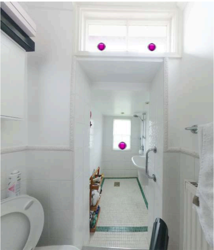
First Floor Bathroom: see high level window dissected by rear extension, and low ceiling in shower area
