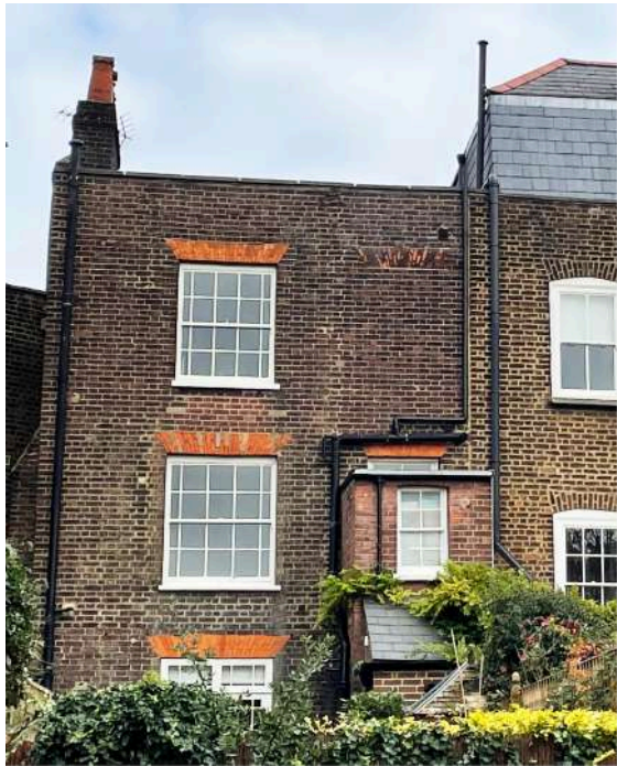
View of 3 Holly Mount Rear Elevation, from Mount Vernon: Evidence of Bricked in Window on the Second Floor, and the later Extensions. Showing the construction of extensions over 1st Floor Window at right hand side
