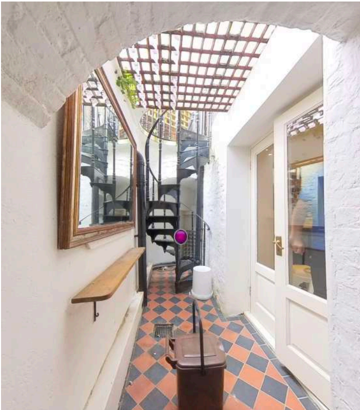
Existing Rear Areaway, see cast Iron Staircase and grating to be preserved with the creation of a new lobby
