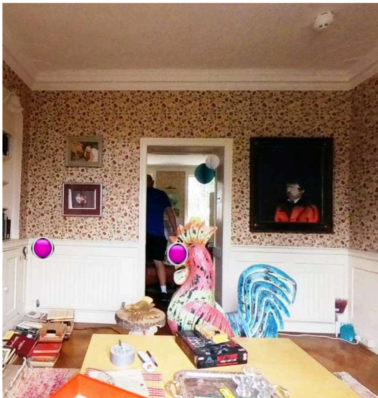
Ground Floor Drawing Room looking to Living Room: see opening to be widened, preserving all plaster mouldings, coving, and cornicing, see non historic herringbone laminate flooring to be replaced
