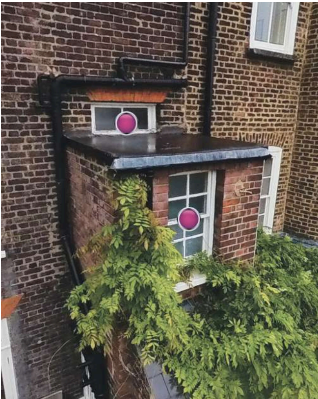
Existing Rear Extension: top windows dissected by roof, lower window with incomplete and obscured arch
