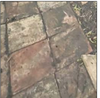
Existing terracotta tiles
